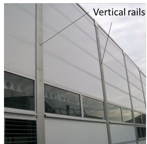
Figure 10. Structure incorporating panels mounted using vertical guide rails.
